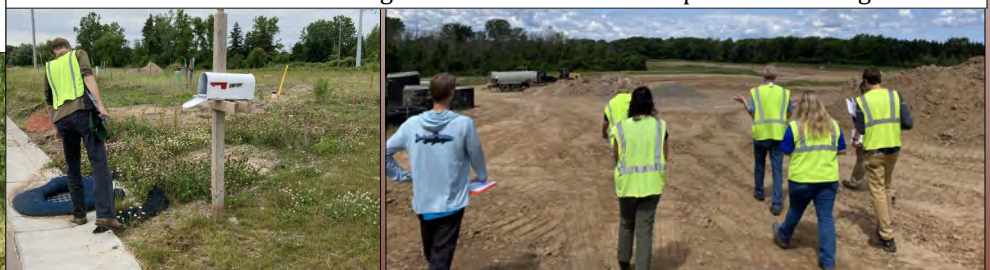
District staff conducting In-Field Construction Inspection Training
