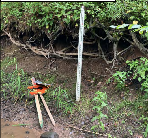
Severe erosion undercutting a tree along a streambank
