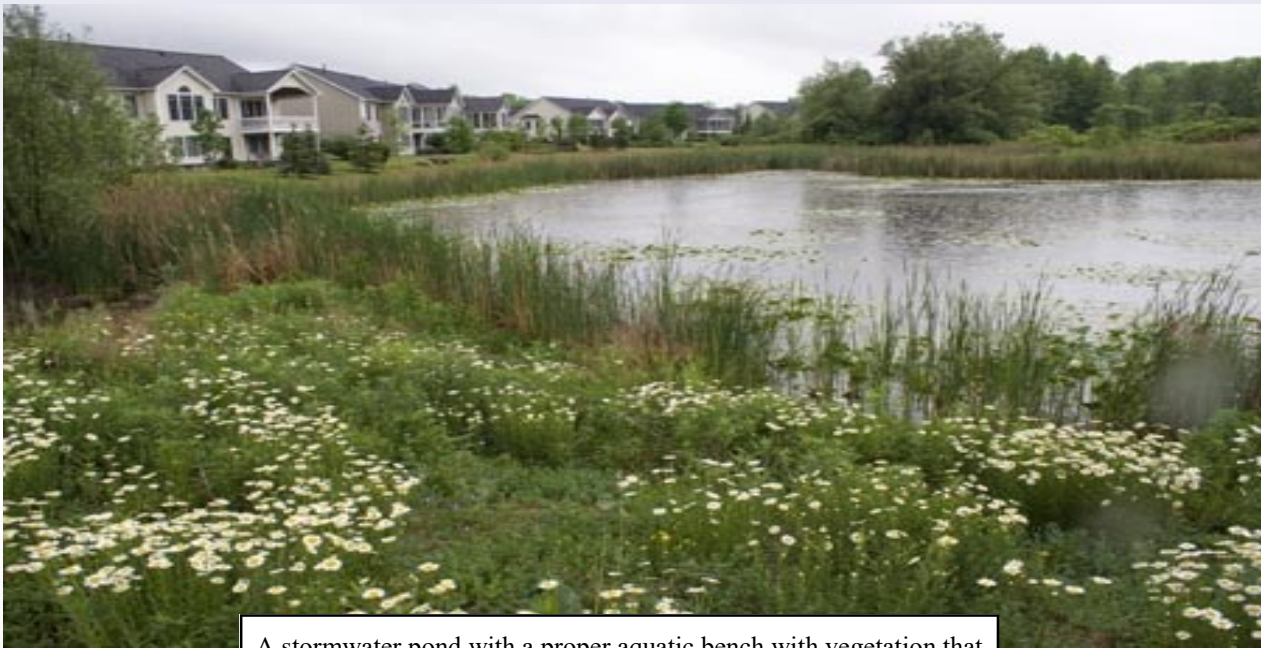
A stormwater pond with a proper aquatic bench with vegetation that provides treatment for nutrients
